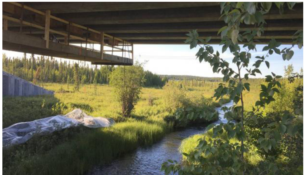
A new bridge over the East Fork of the Moose River will provide a more natural wildlife underpass after the existing small culvert and roadbed are removed. Photo by John Morton
