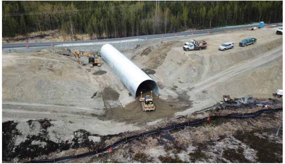
An aerial photo of the longest of five culverts being installed under the Sterling Highway. Photo by Shaun Combs, DOT&PF.
